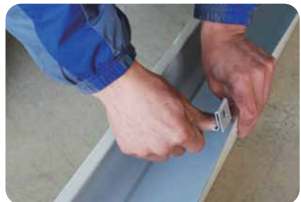
Gutter Hook Installation
