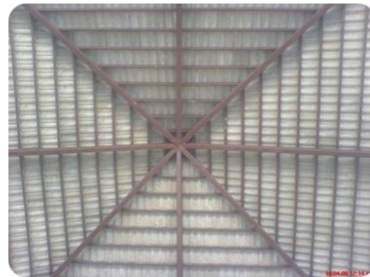
Open structure, underneath of the IGNC A open roof
