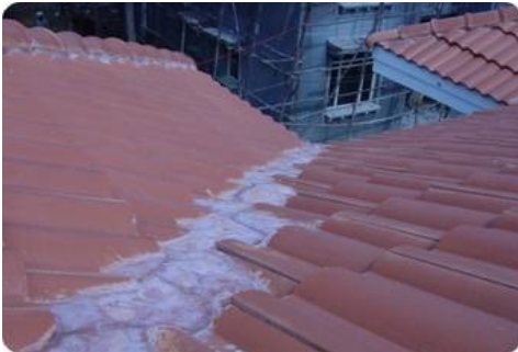
Conventional way....with mortar
