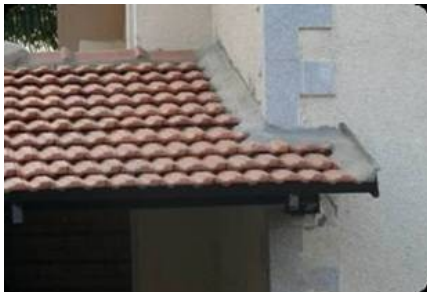
Conventional way....with mortar
